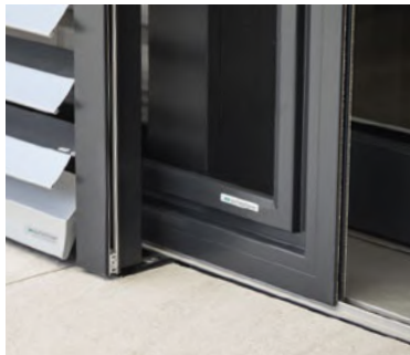
Self-supporting guiding rail for sliding frame of insect protection
